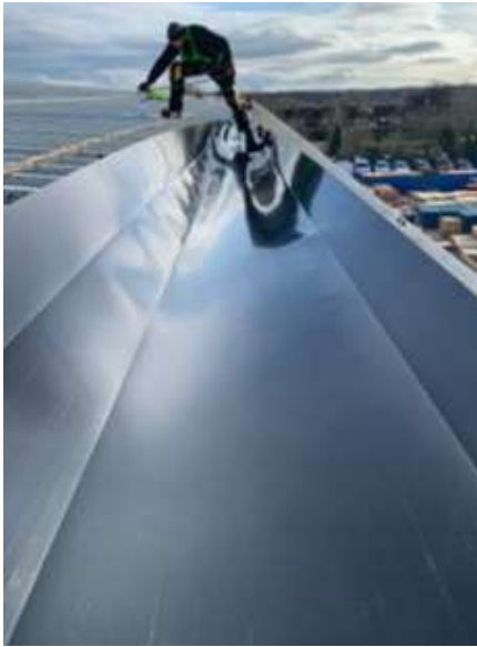
Gutter Lining
