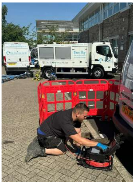
CCTV Drainage Inspection
